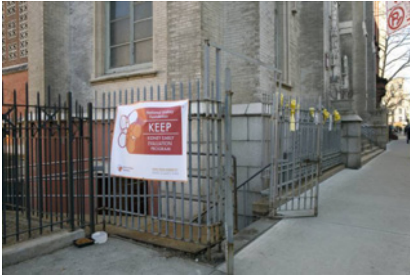
St. Charles Borromeo Church 211 West 141st Street, New York, NY 10030
